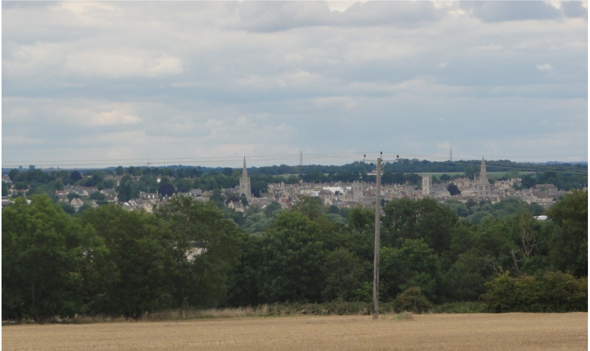
Figure 26: View of Stamford town centre from south-west (Macmillan Way at Easton-on-the-Hill). The western half of Area 2 is visible as the higher land on the right of the picture, forming a green backdrop to the town. Note also Area 4 (between viewpoint and Stamford town centre) is screened from here (see Area 4 text)
