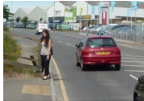
Poor footway facilities on Gonerby Road
