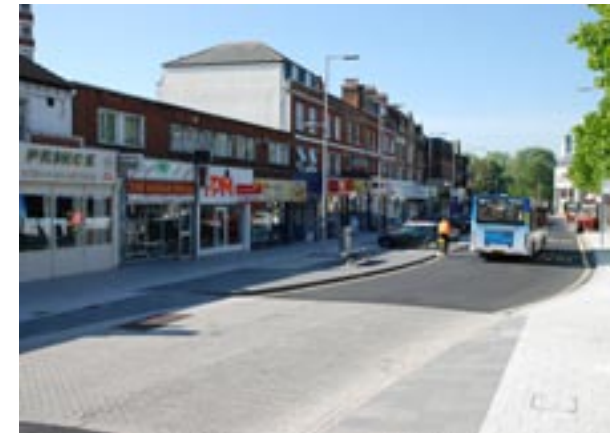
An example from London Road, Southampton where traffic speeds have been reduced significantly through the use of raised tables.
