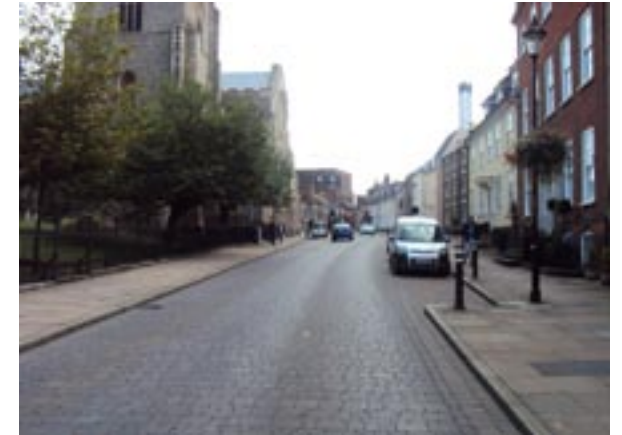
Street improvements have transformed the quality of the historic urban streets in Bury-St-Edmunds
