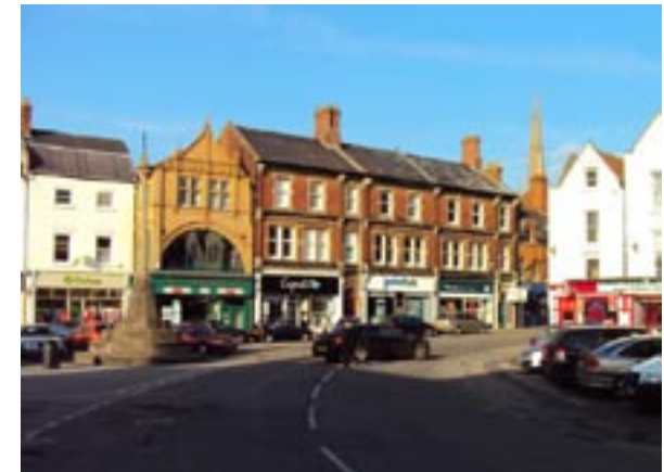
The link to the High Street shown will be transformed into a pedestrianised link
