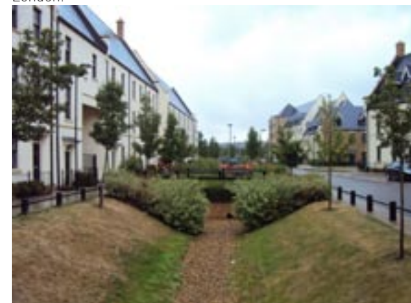
Upton, Northampton illustrates how a SUDS network can be integrated into the street pattern, as is proposed for the Poplar Farm development.
