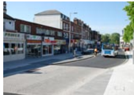
Example of a well designed raised table on London Road, Northampton
