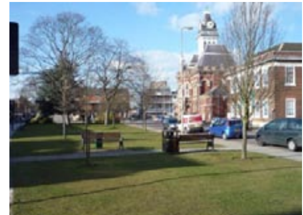
The St Peters Hill service lane will be designed as an extension to the park
