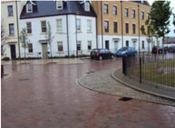
Upton, Northampton has delivered high quality public realm improvements and new open spaces as part of its medium density housing offer
