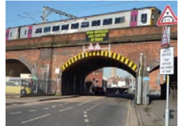
The Victorian rail embankment limits east west connections in Grantham
