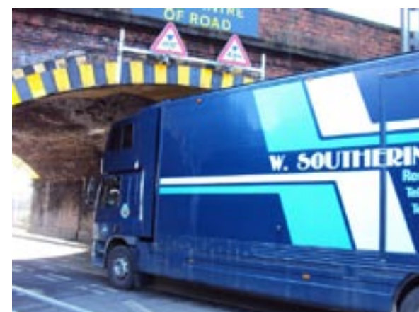
Low bridges mean that freight has to use the centre of the carriageway to get under them.
