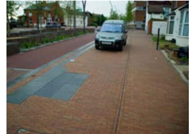
The delivery of more shared street layouts that encourage use of space for a variety of vehicular and non-vehicular modes in Ashford.
