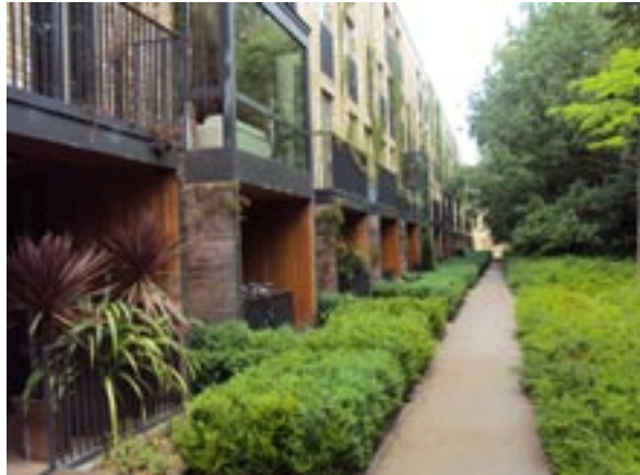
High quality architecture and the integration of a natural water course throughout Accordia gives it its own sense of place and identity.
